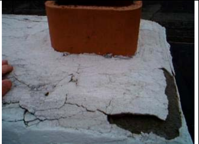
Deterioration on chimney crown
