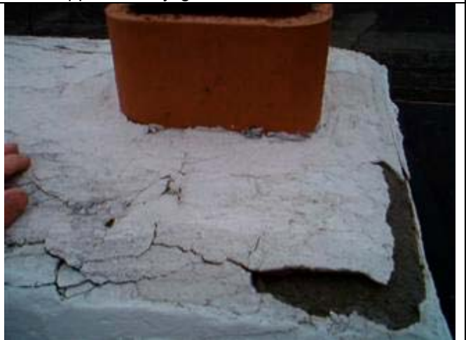
Deterioration on chimney crown
