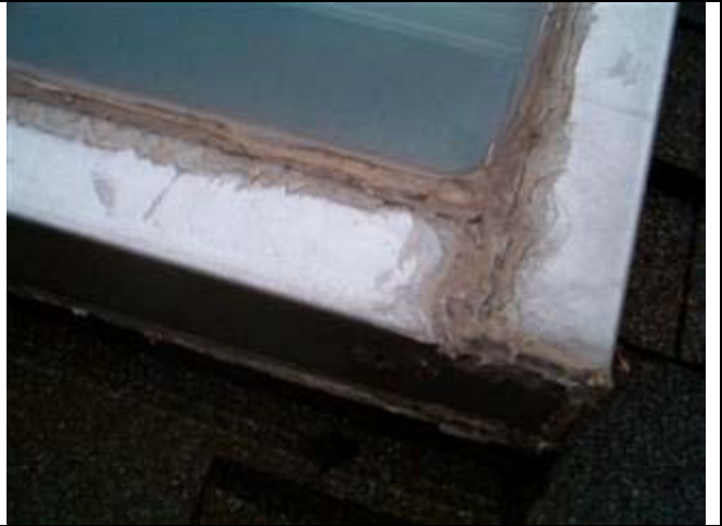
Caulk applied to skylight
