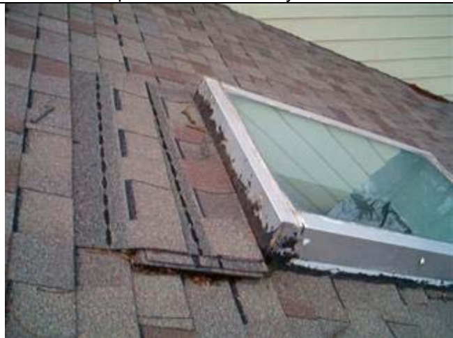
Shingles piled above skylight
